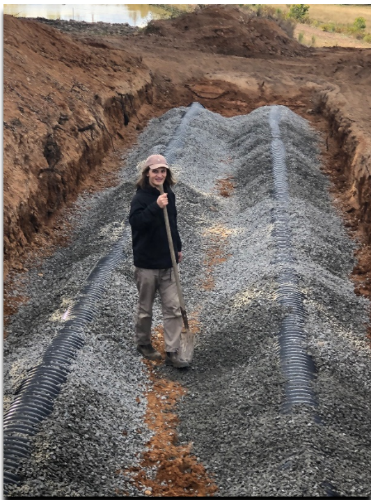
Tom Toparis helping install drainage pipes
