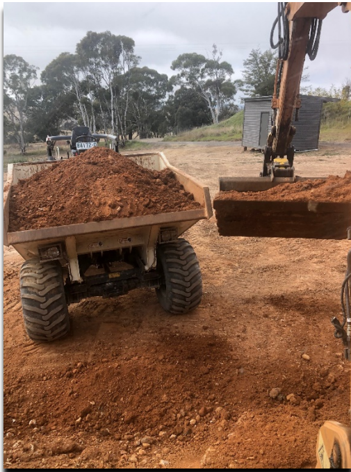
Track material being loaded
