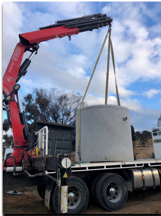
Septic system being installed
