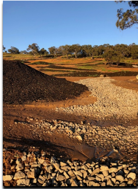
Drainage and water runoff works
