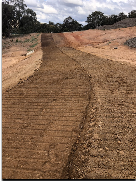
Track surface after tiller prep
