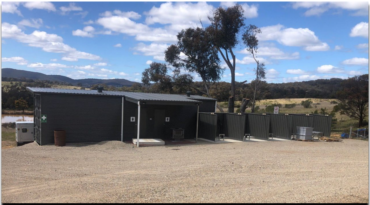
Amenities and washdown bays
