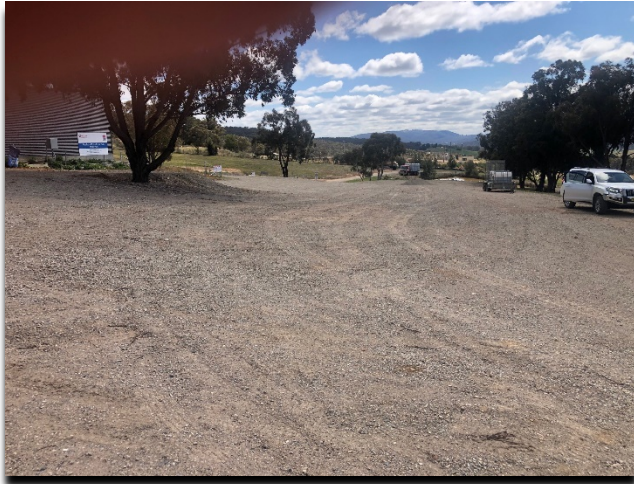
Pit area and car park construction
